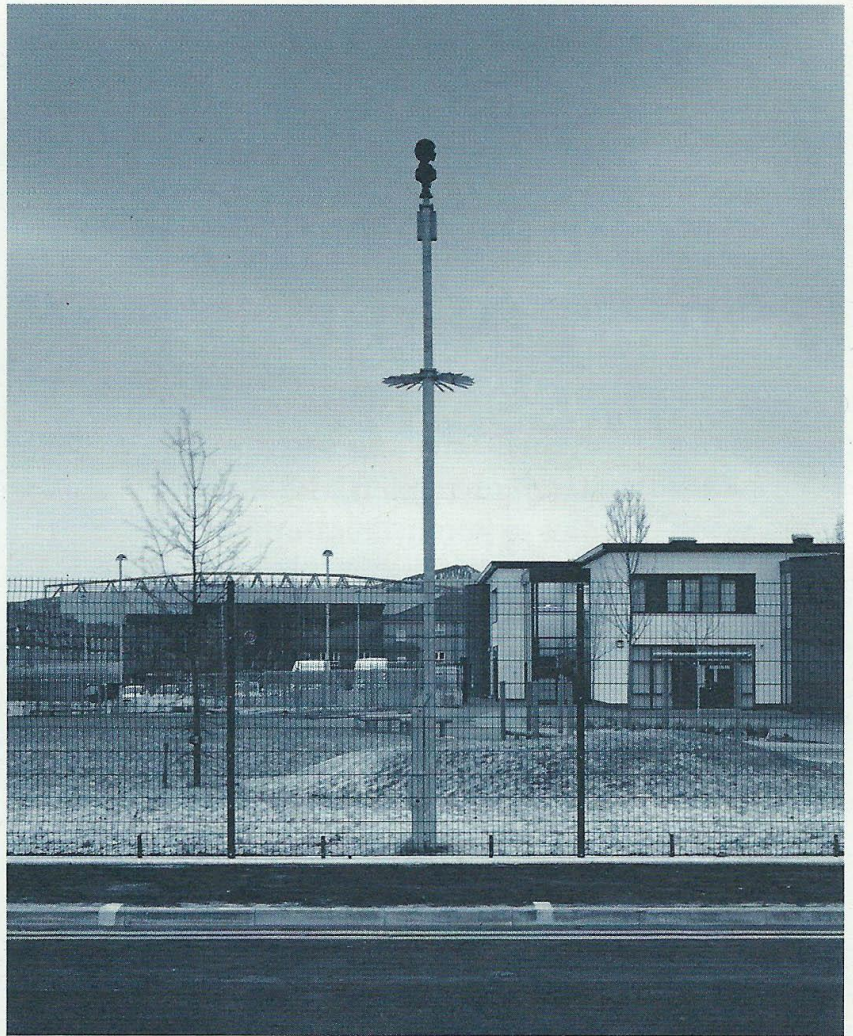
High-security fence factory, 2012.
