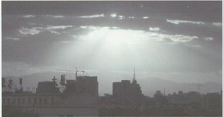
Works for the New Library, Renmin University Campus, Beijing, 2009. Photo by Olivia Bina.
