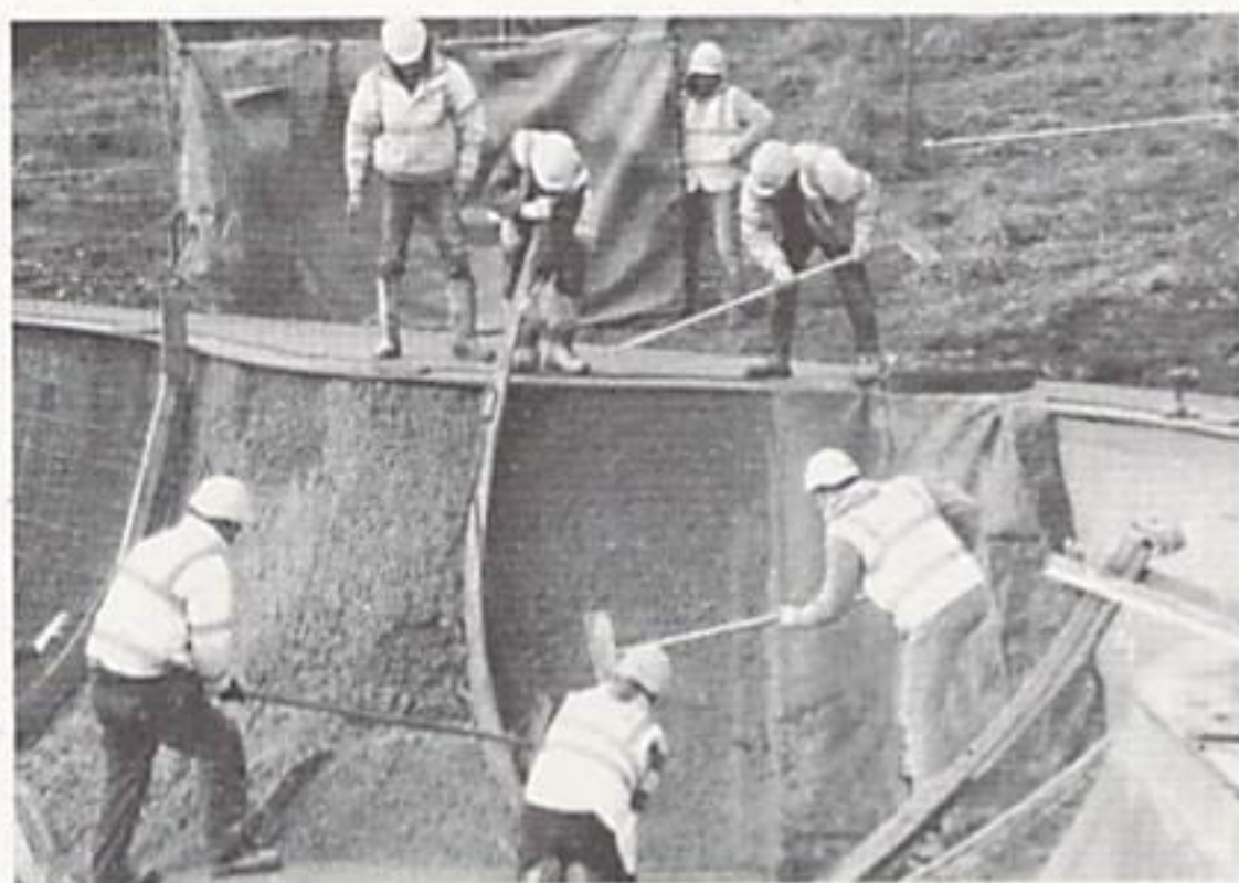
Pool construction by Canvas, November 2017. Photo by Iain Borden.
